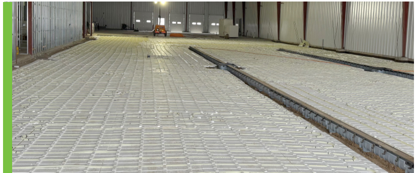
Radiant Results: Inside the warehouse, GeoStar water-to-water systems power radiant floor heating, ensuring consistent warmth despite South Dakota's frigid winters.
