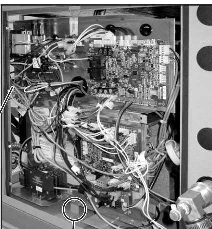
Figure 13b: Wire access (control box closed)
