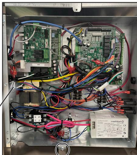
Ground Fastener must be installed for proper unit ground
