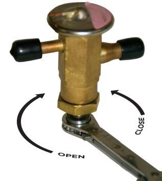
Figure 4: Decrease Superheat: Open Valve Increase Superheat: Close Valve
