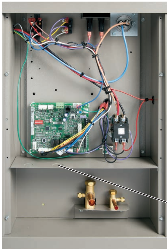
Figure 13A: Wire access (control box open)
